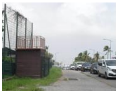
Station trafic BOUCHON
